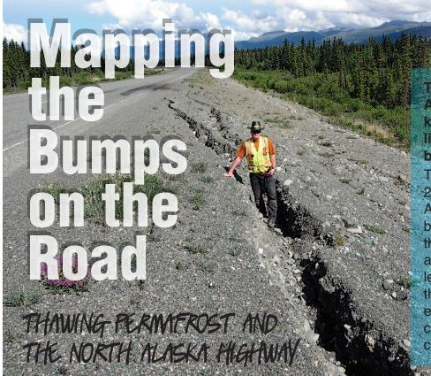
**Travelers** of the **Alaska Highway** know what it is like to drive a bumpy road. The northern 200km of the Alaska Highway is built on permafrost that is thawing and becoming less stable due to the combined effects of construction and climate change.
