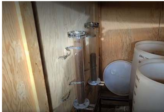
Figure 4: Columns C1 and C1b installed in series of BR1 and BR1b in the onsite research shed.
